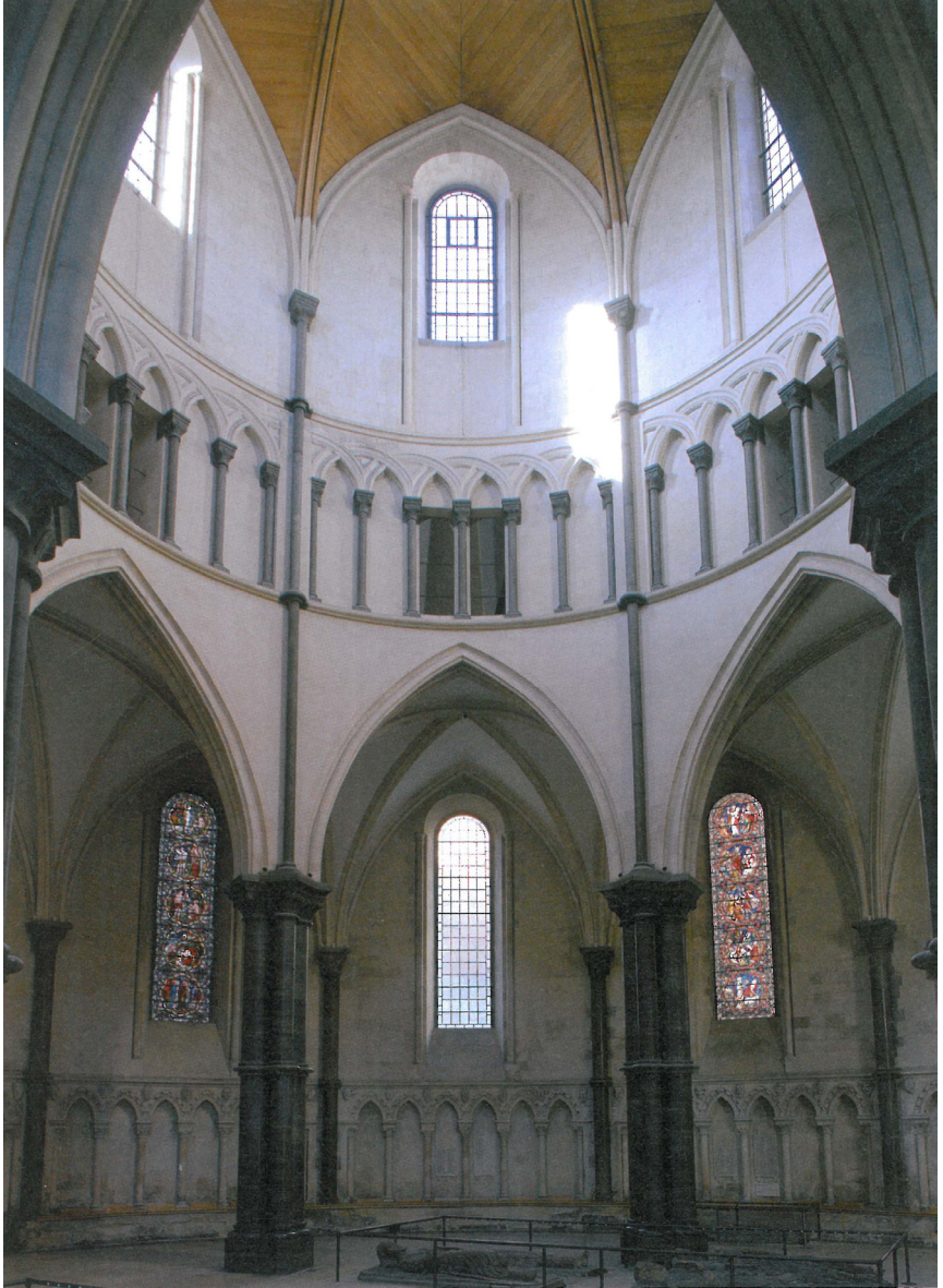
Figure 4. The interior of the round nave of the Temple Church with arcade, gallery and clerestory. Photo: Øystein Ekroll.
